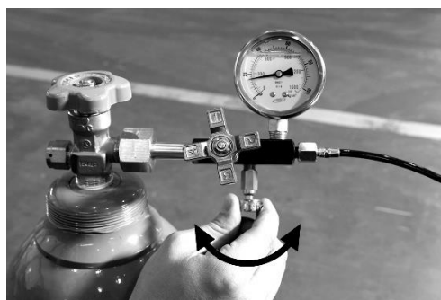
10. Drain the gas to 55~60 kg/cm 2 upon ambient temperature of job site.
